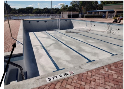
new finished pool w coping removed creating a flat edge for pool entry
