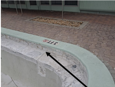
Cracks in coping (edge)
